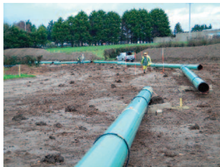
Steel pipeline laid out along the route, ready for welding.
