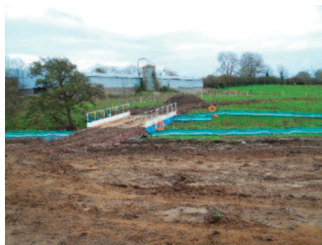
Bailey bridge silt fencing to protect waterway.
